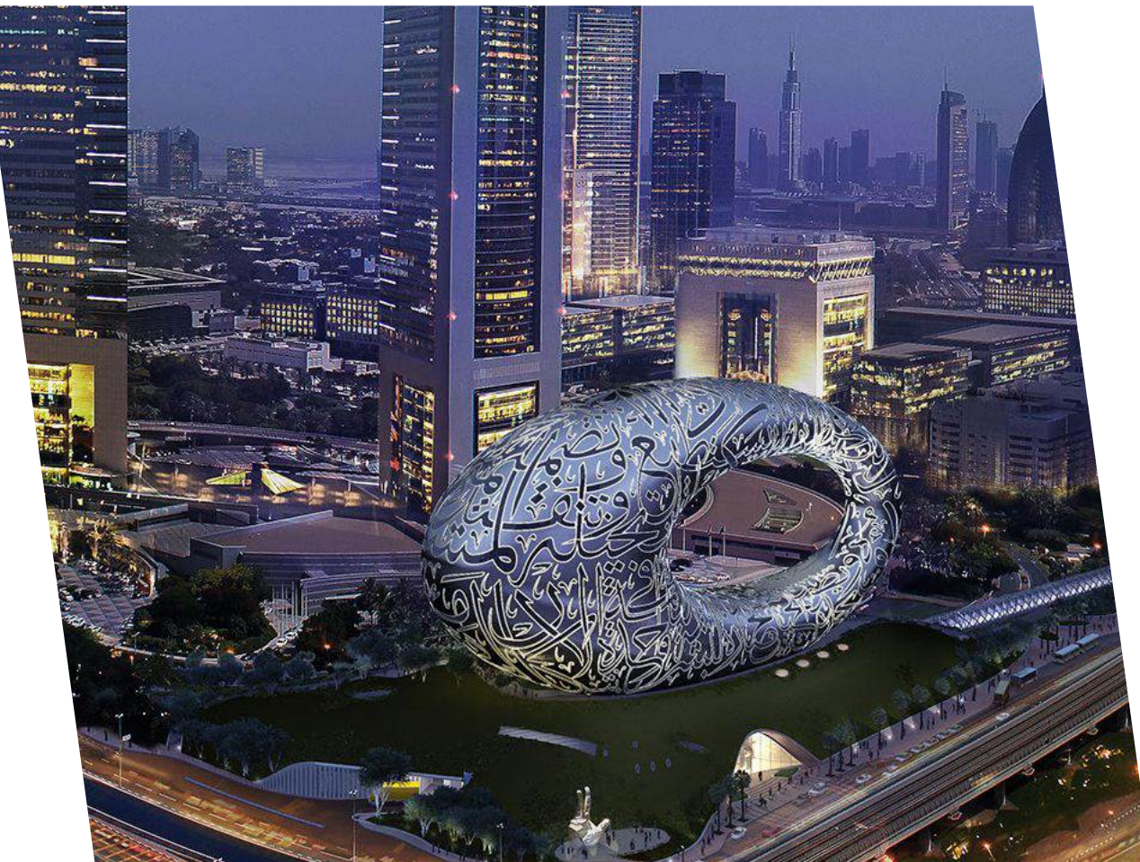
The museum’s futuristic facade features windows engineered into calligraphy forms. Courtesy of Killa Design.
