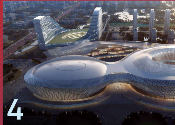
4 A Green BIM Process Shapes Construction of an Iconic Sports Venue in China
