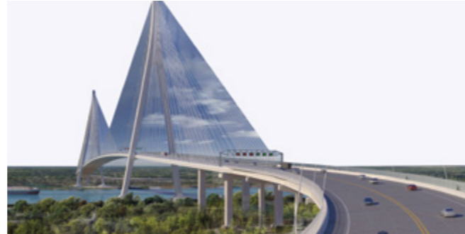
Gordie Howe International Bridge
