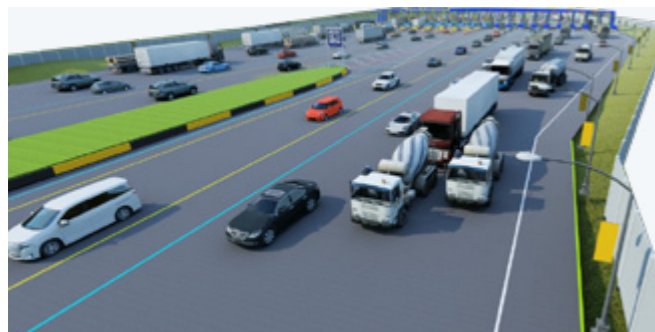
Manado Bitung Toll Road Project PT PP (PERSERO) TBK, Indonesia
