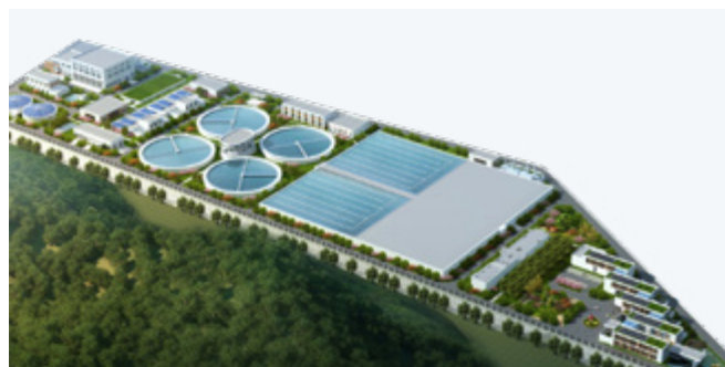
Jiangxia Sewage Treatment Plant
