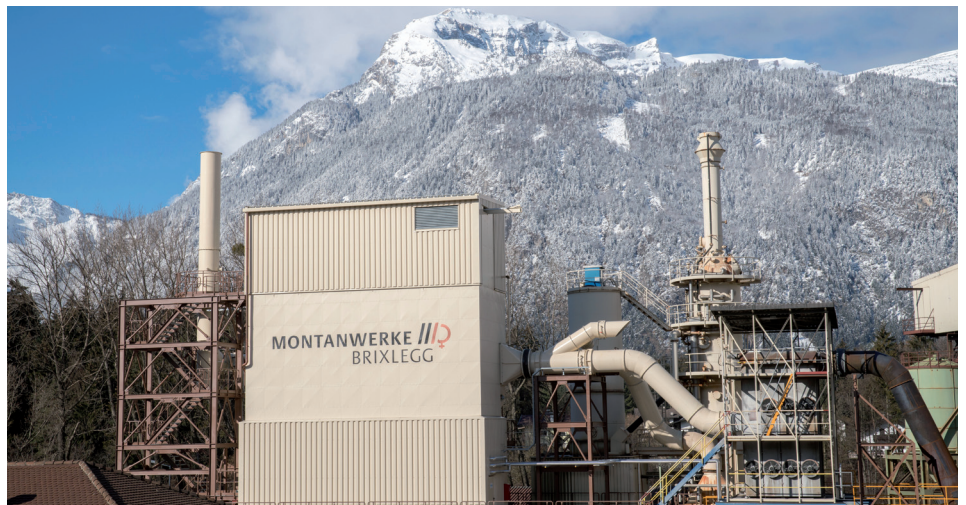
Also in the mining works in Brixlegg / Austria Scheuch proved itself as a competent problem solver with a modern kiln dedusting. © Scheuch GmbH
